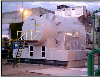
Fig. 3. CPAV01, synchronous compensator of Vila do Conde substation-PA.
